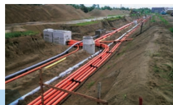
地中送電線路工事 Buried Transmission Line Construction
