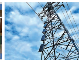
山間部ネットワーク装置 (携帯圏外エリアで活用) Mountainous Area Network Facility (For areas outside mobile phone coverage)
