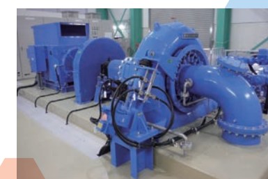
木本小水力発電所(発電事業)水車発電機 Konomoto Small Hydroelectric Power Station (Power Generation Business) Hydraulic Turbine Generator
