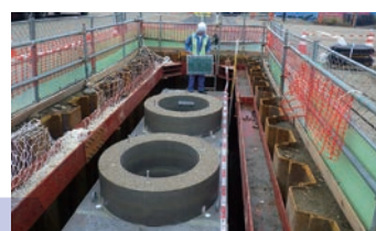
地中送電線マンホール据付工事 Buried Transmission Line Manhole Installation Work
