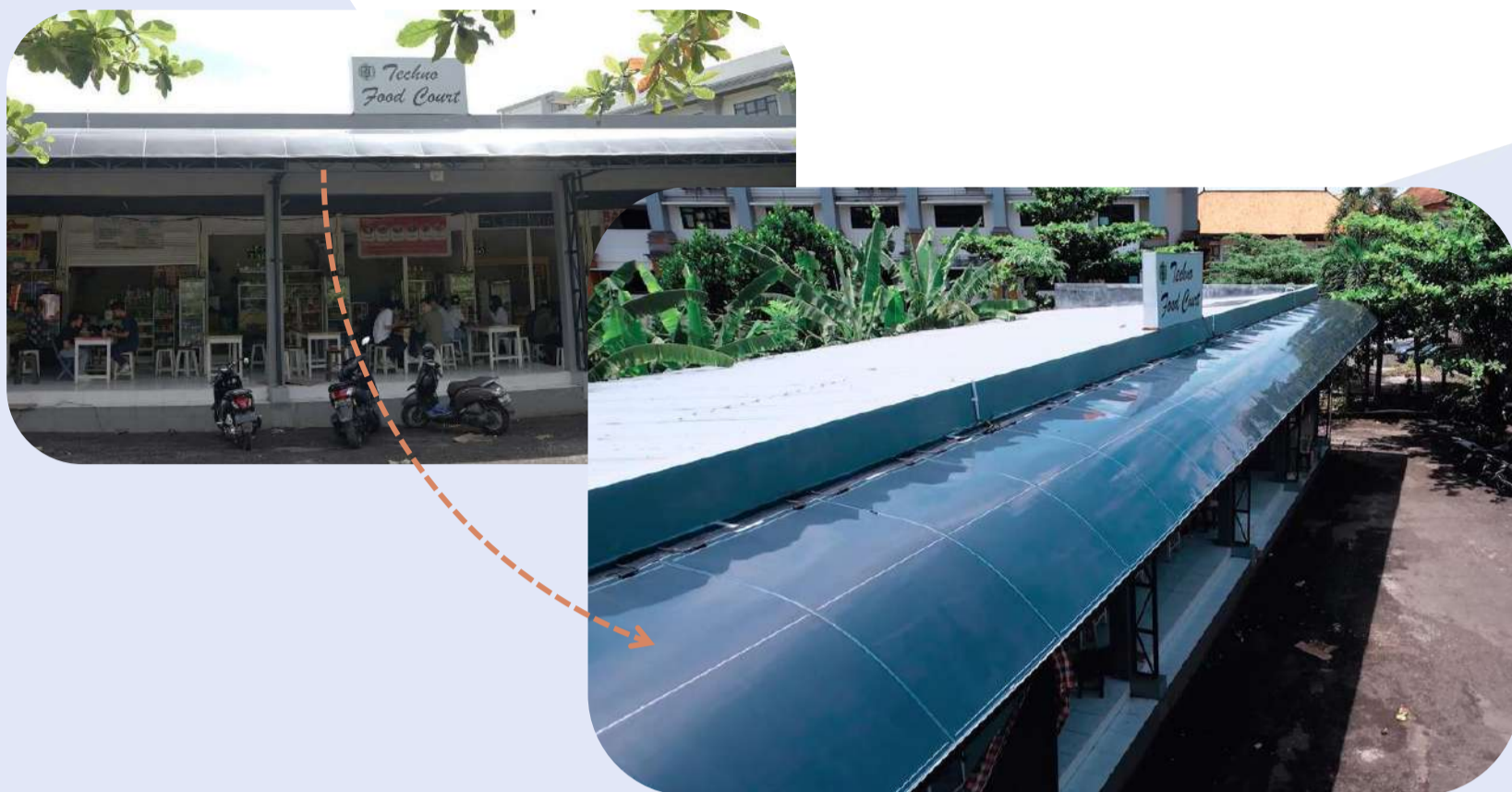
Flexible Solar Panel Installation at the Canteen of Engineering Faculty of Udayana University
